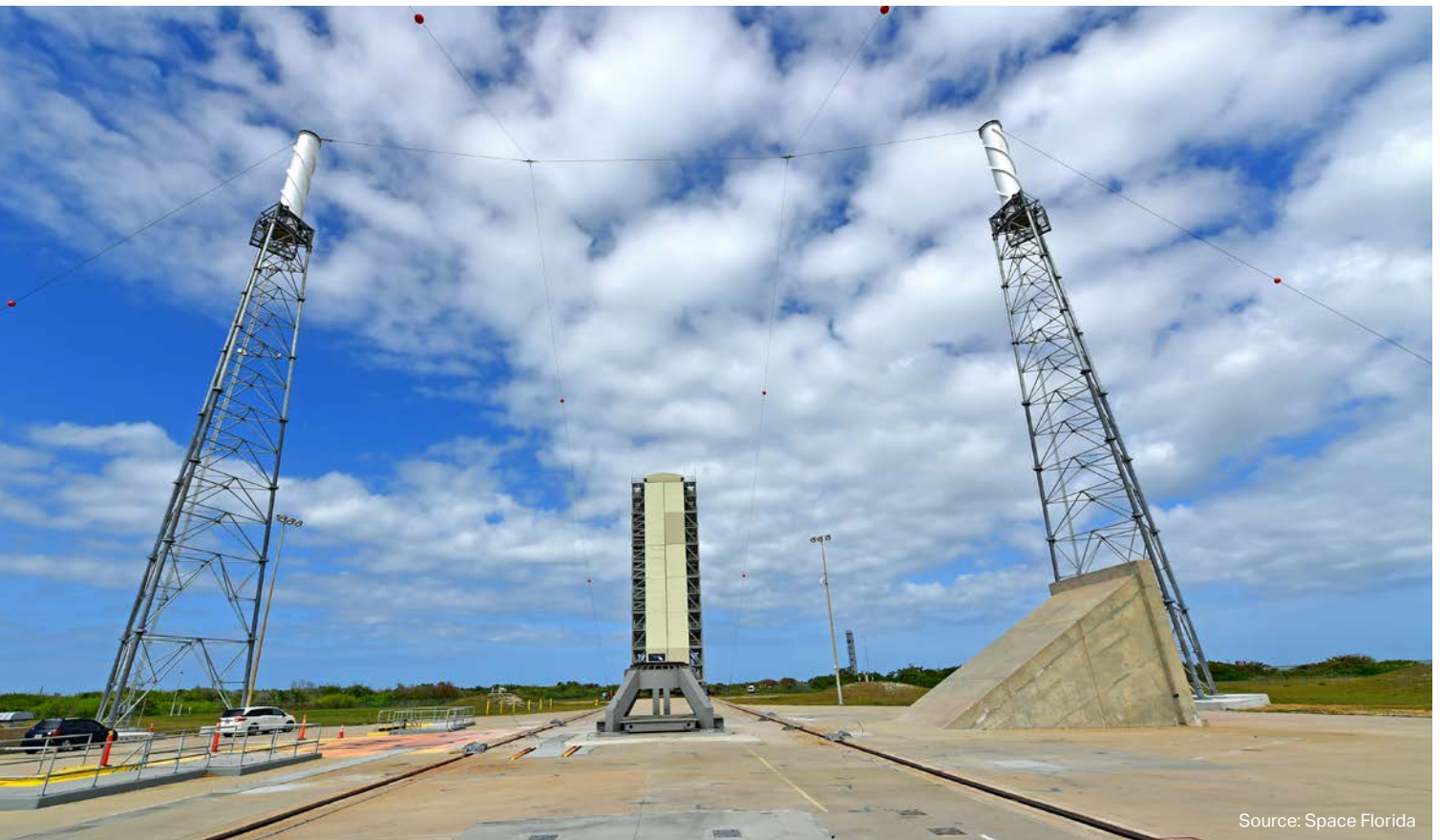
Launch Complex 46 Mobile Access Structure, flame duct, and lightning towers
